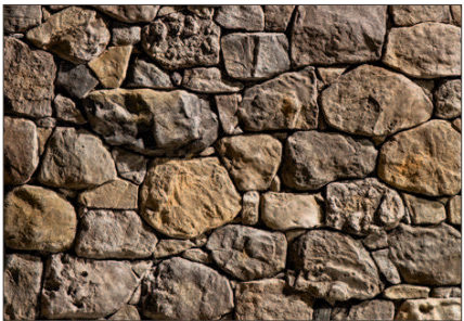
dry-stack joint
