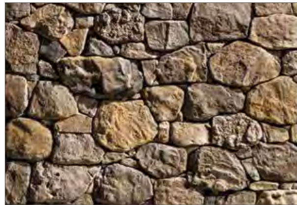
dry-stack joint
